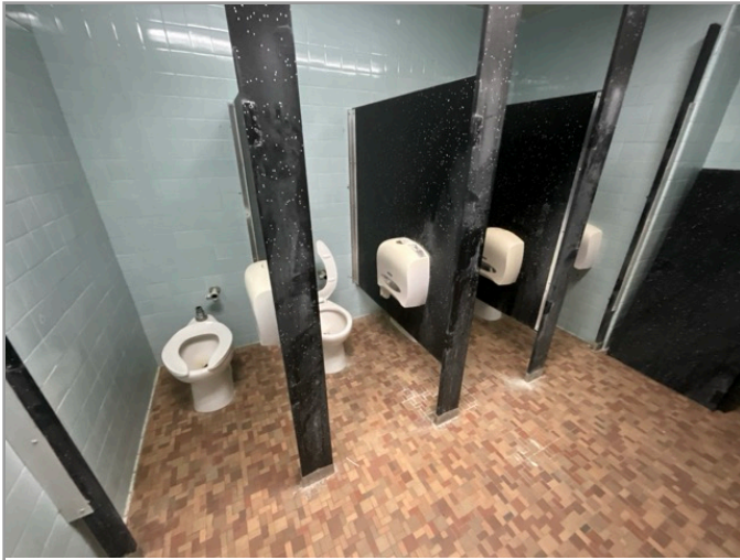
TOILET STALL OVERVIEW
