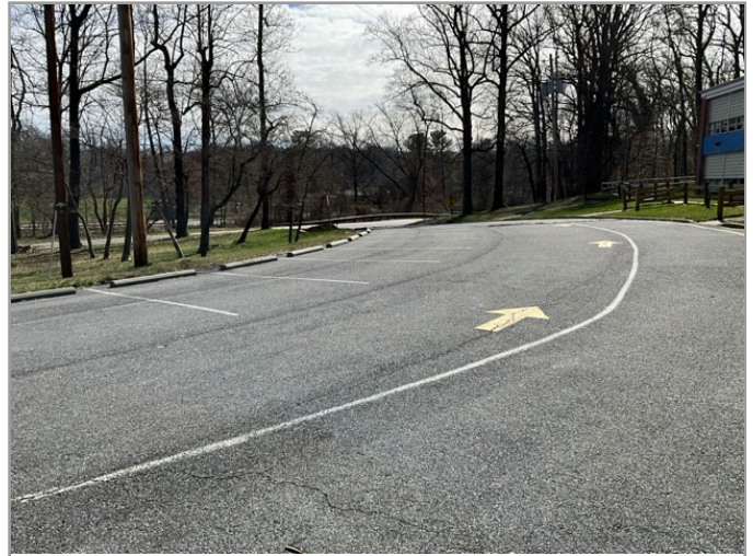
NO ADA PARKING OBSERVED
