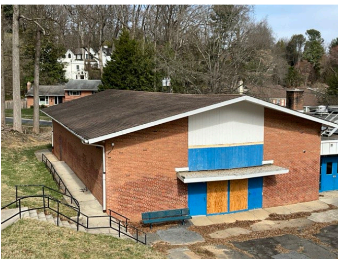
5 - ASPHALT SHINGLE ROOFING
