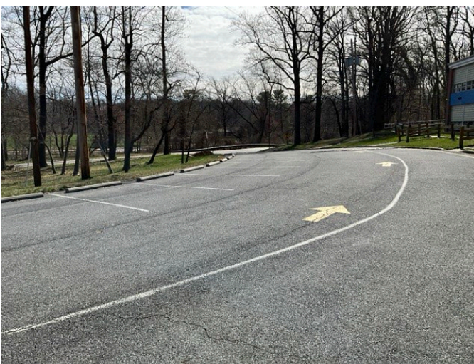
23 - PARKING LOT OVERVIEW
