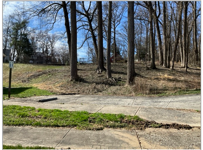
NO ACCESSIBLE ROUTE TO PLAYGROUND
